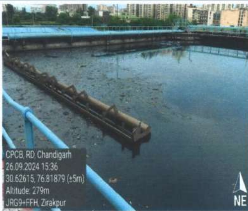
View of Floating Plastic Material in SBR Tank of STP.
