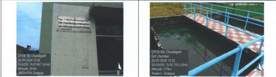
View of 17.3 MLD STP of Zirakpur.
